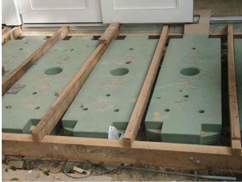
Figure 26 - Flat water storage. Hard plastic water containers to be stored under porch, patio or deck.
