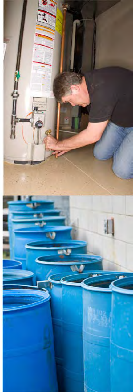
Figure 24 - Water storage. Top: Using water from your water heater. Bottom: 55-gallon food grade water barrels.
